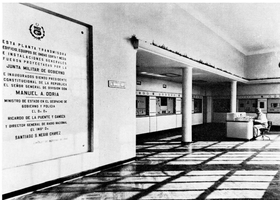
50 kW short-wave and 20 kW medium-wave broadcast installations at Lima, Peru.
