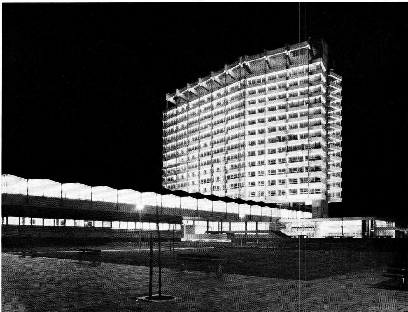
Floodlighting by 150 iodine lamps 1000 W of the new office of Philips Nederland n.v. at Eindhoven. In addition the building has windowlighting by "TL" fluorescent lamps.
