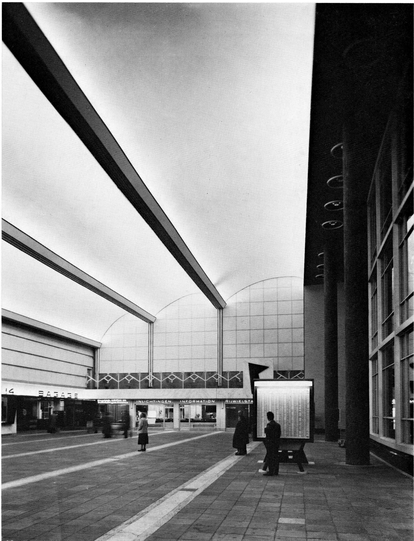
Indirect lighting of "TL" lamps in the hall of a railway station.
