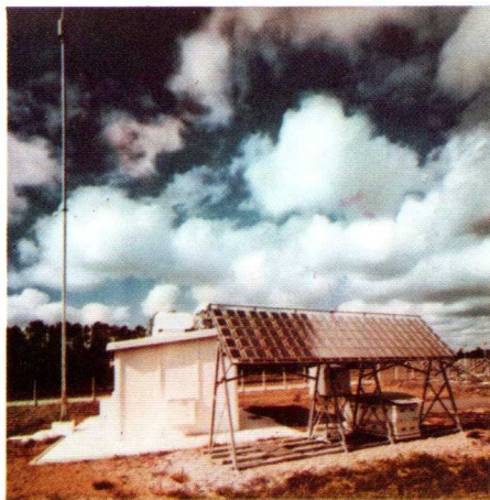
Permanent 50W power generator station for radio beacon near Saint-Girons in the south of France, some 30km from the Spanish border. ▶
